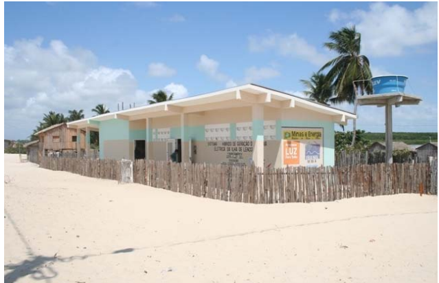
Figure 10: Control & power house
